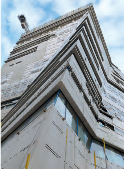
The superstructure for the new Tate Modern reached its full height
