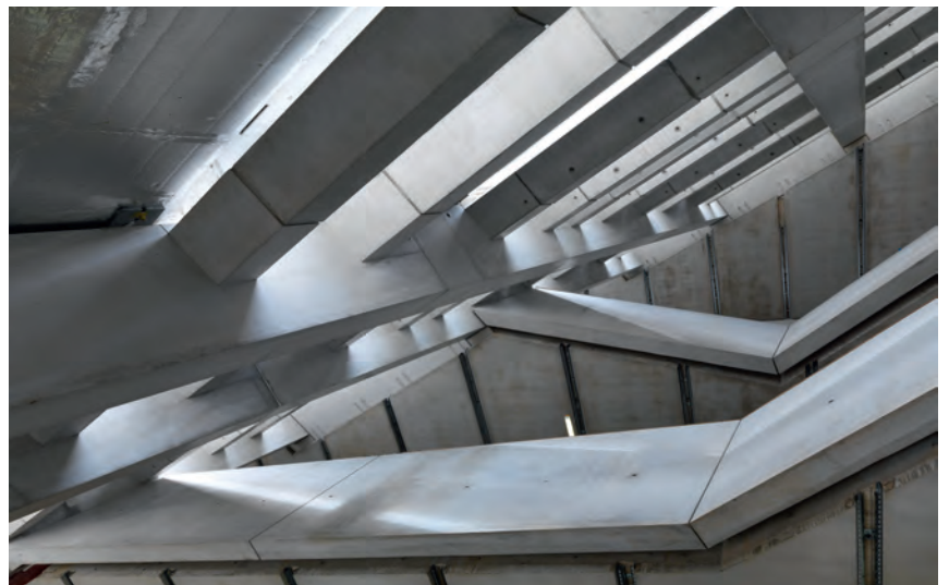
The interior of the new building uses raw concrete folded into complex angles and shapes
